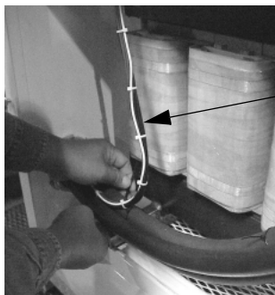
Figure 3-13 Tie-wraps on the AC Sense Harness
